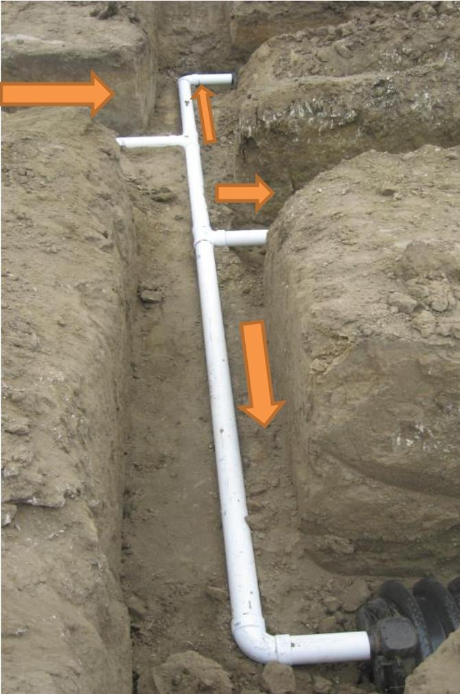
Trenches are to be no deeper than 48" to the bottom with at least 12" of soil over the top.
