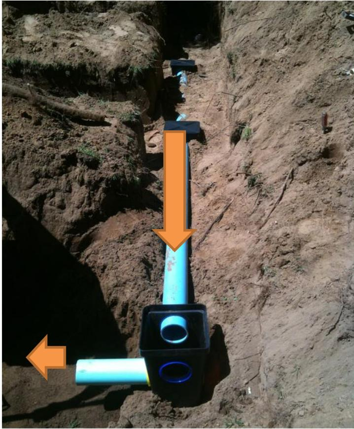
Distributes the effluent from the septic tank to an absorption field located on slopes.
