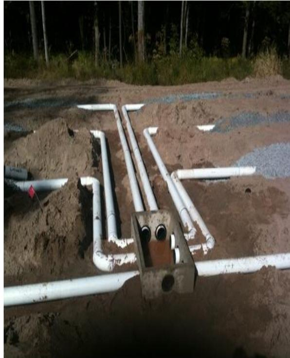
Distributes the effluent from the septic tank evenly to the absorption field or seepage pits. It is important that each trench or pit receive an equal amount of flow. This prevents overloading of one part of the system.
